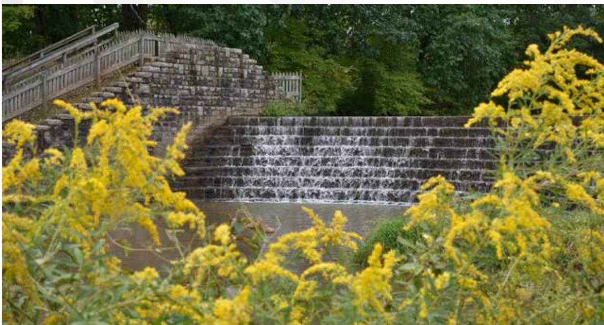
The Boone House, opposite, and the dam at Daniel Boone Lake, above, at Daniel Boone Homestead in Birdsboro. Photos, PHMC
